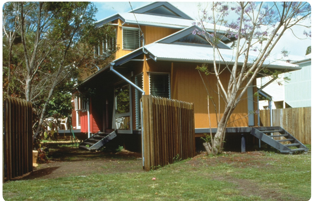
Large overhangs provide good protection.
