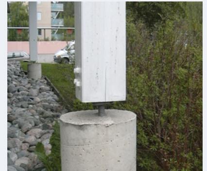
A well-ventilated, free-draining post support.
