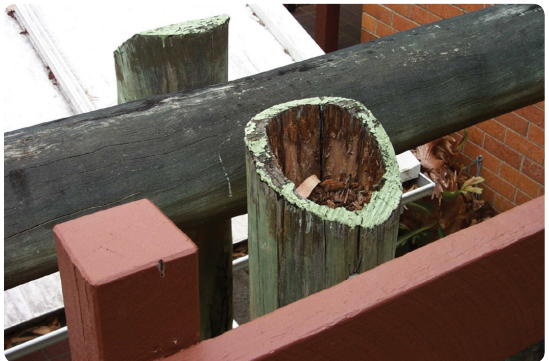
CCA treated sapwood outperforming durability class 2 heartwood
