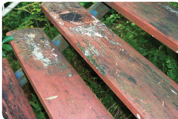
Poor maintenance of stair tread.
