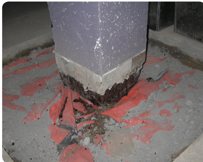
Degradation of basement column after 100 years in service in Brisbane.
