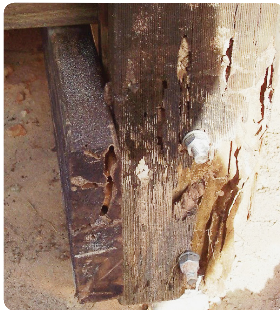
Termite damage to non-resistant timber.
