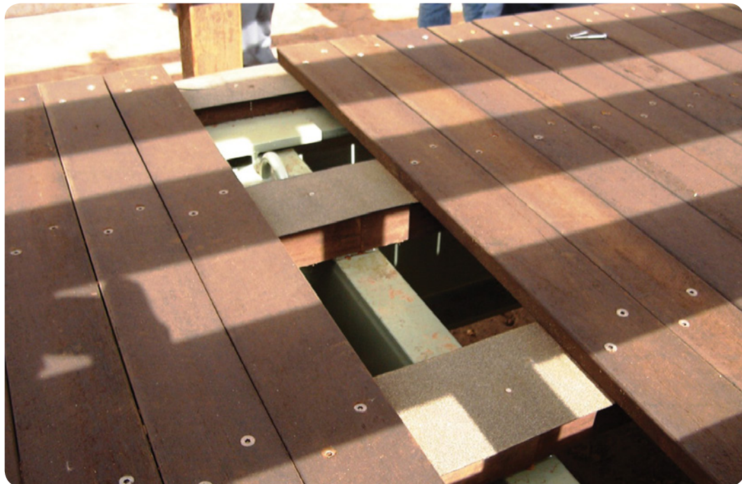
Good detailing (staggered screws and DPC over joists) used for this prefabricated bridge.
