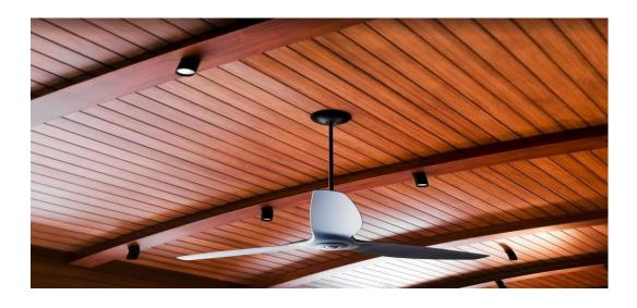
Timber lining is kiln dried to an average moisture content of 9-14%, which is suitable for internal use.
